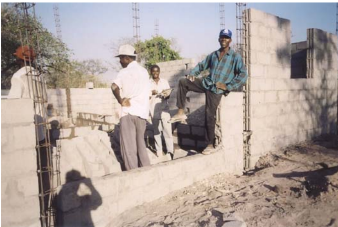
Building labourers working on the new health centre
